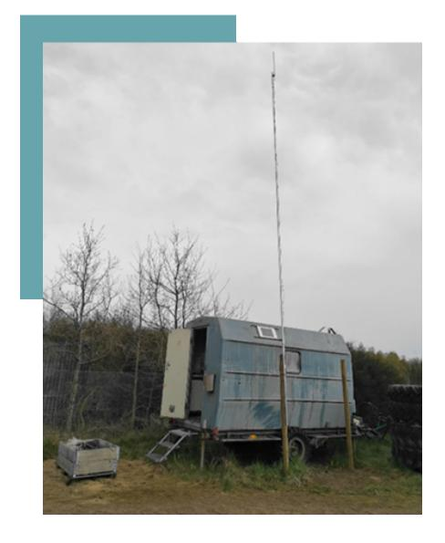
When selecting the location for the high-gain antenna/Base unit consider that you will mostly control irrigation from the app. Thus placing the Base closer to the valves (or pump) is better than placing it closer to your home/office.
